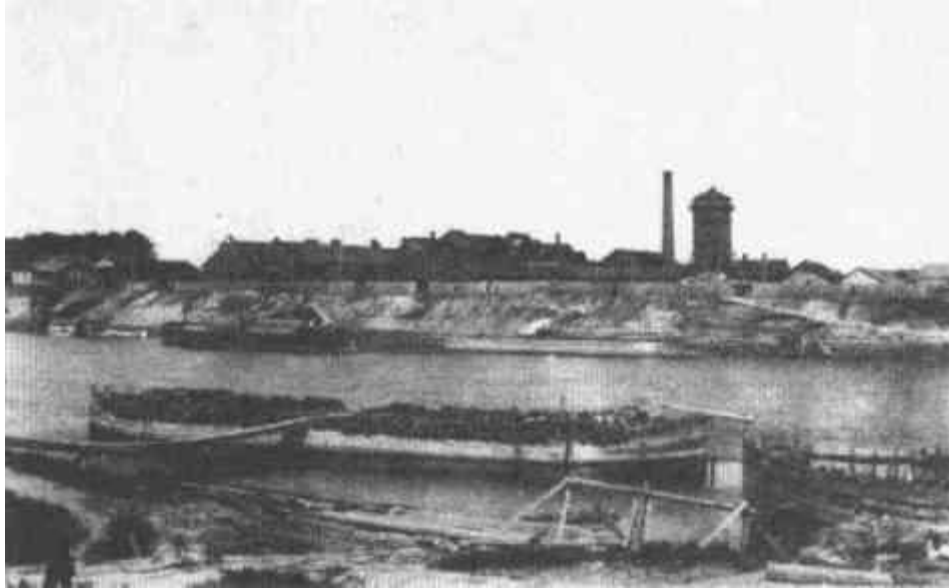
Figure 1. Sokol Paper Mill. The Bank of Sukhona River.
