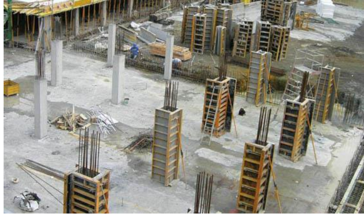
Figure 2. Photograph of the building of a structure made of reinforced concrete 2
