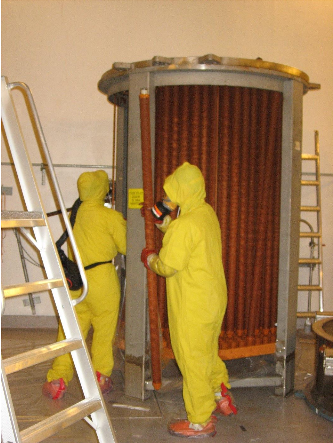
Picture 8 Old rods being removed, during the filter change [Saarimaa, 2010]
