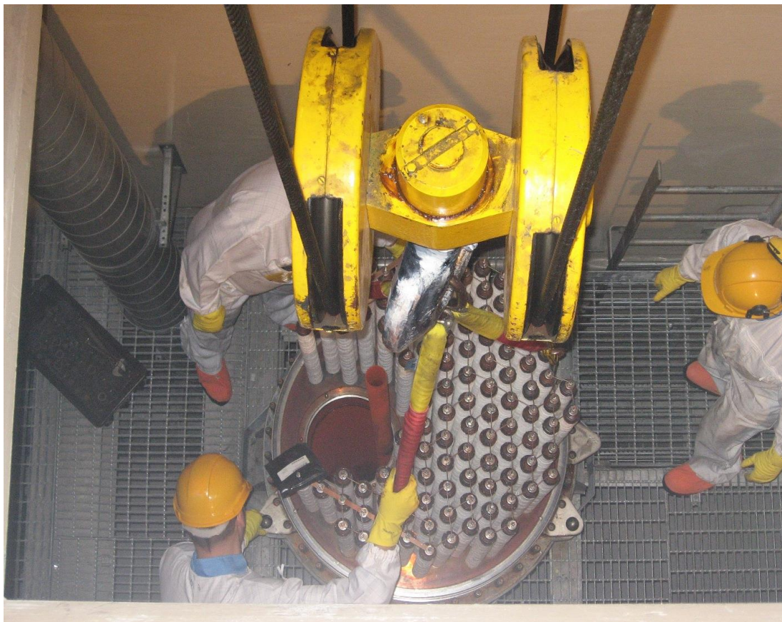
Picture 9 OL2's 332-filter rods being changed in 9.11.2010 [Saarimaa, 2010].
