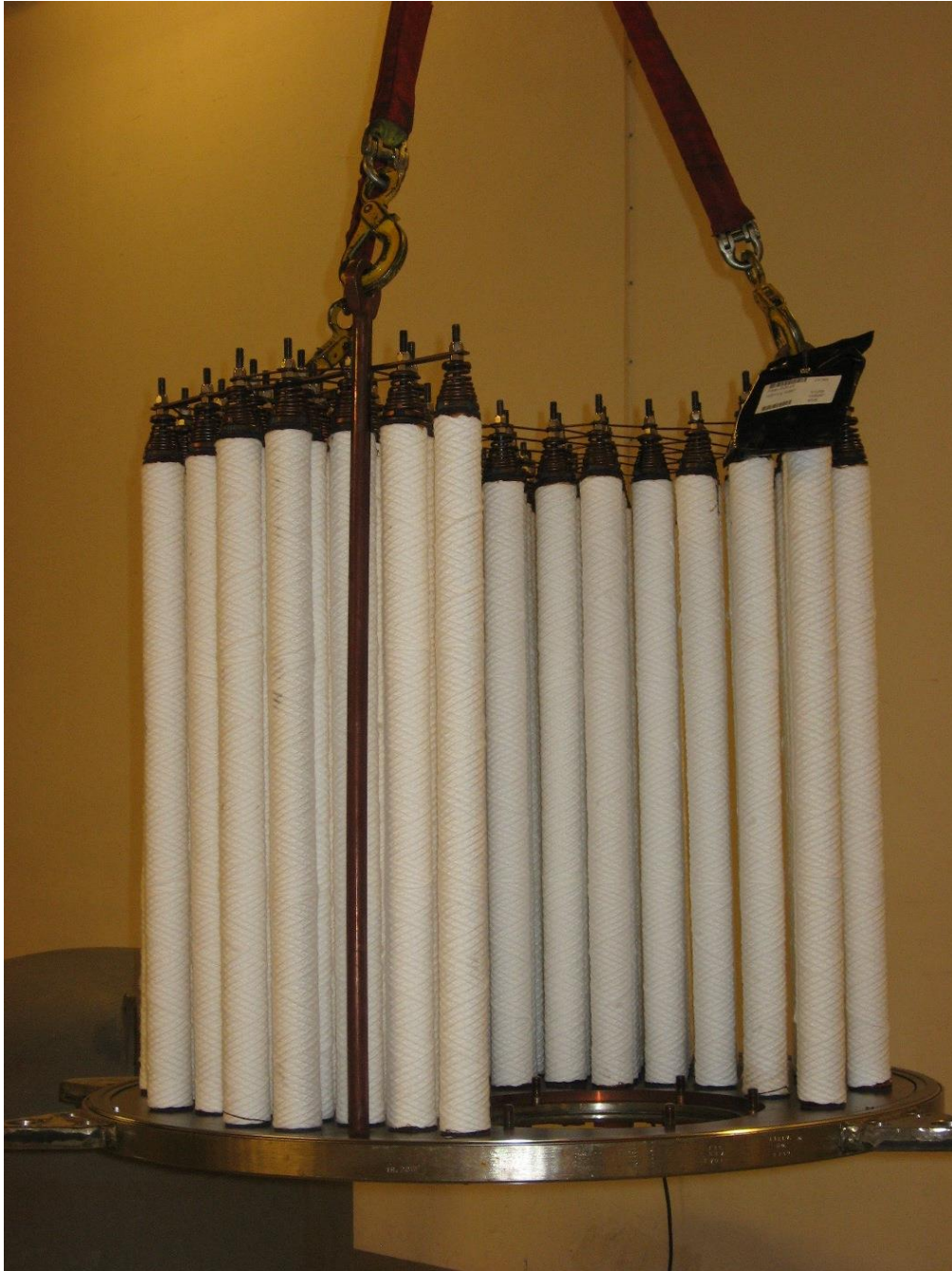
Picture 10 OL2's 332-filter rods being changed in 9.11.2010 [Saarimaa, 2010].
