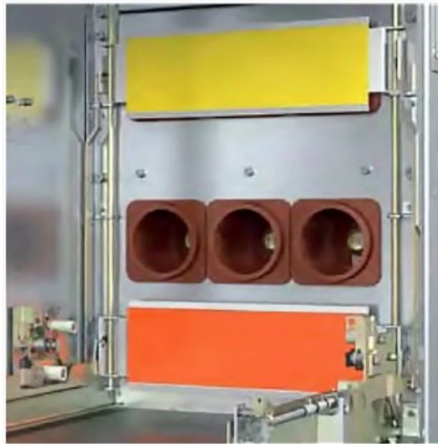
Figure 3 Automatic shutters (Csanyi, Electrical Engineering Portal, 2019b)
