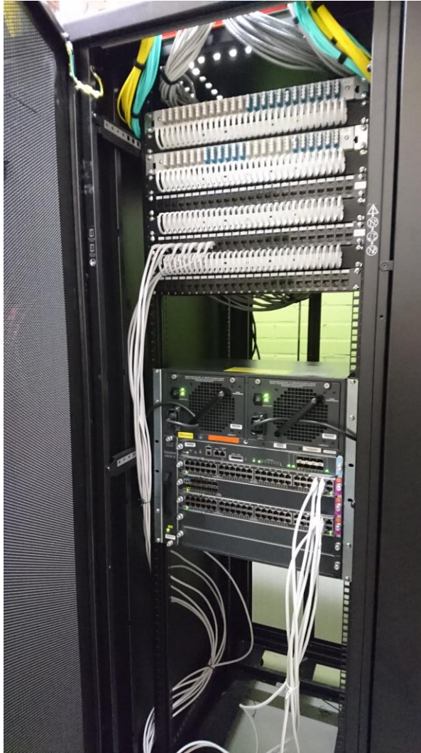
IMAGE 2. Internal rack cabling with a router during initial installation
