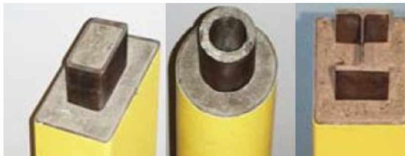
Figure 17. Hollow sections with additional inner profiles
