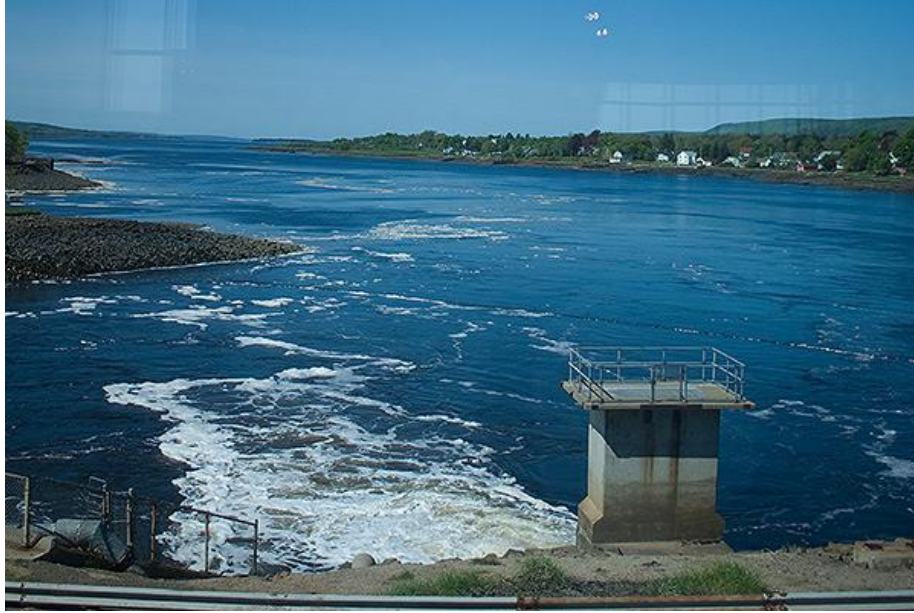
Figure 2 - Annapolis Royal Generating Station, Canada (Source: PowerTechnology)
