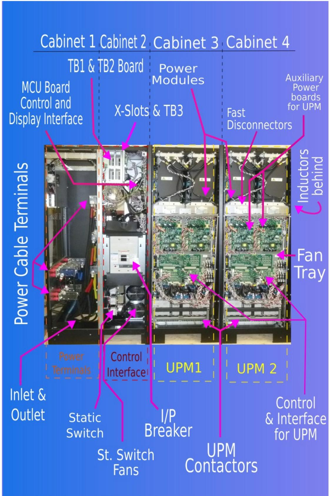
Figure 1. Main components of the UPS unit 9395P sort by cabinets.
