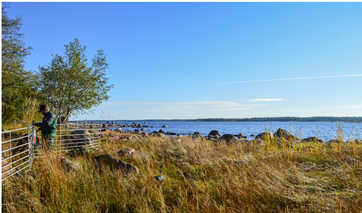
Figure 23. Building the leading fence along the shoreline.
