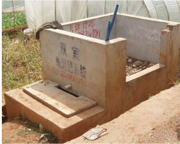
Figure 6-7 The Double Chamber Composting System
