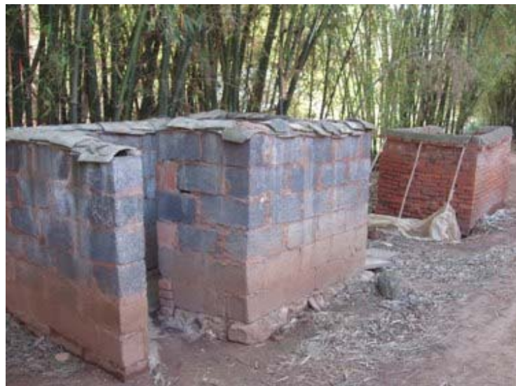
Figure 1-1 Old Toilet (Traditional Dry Toilet)
