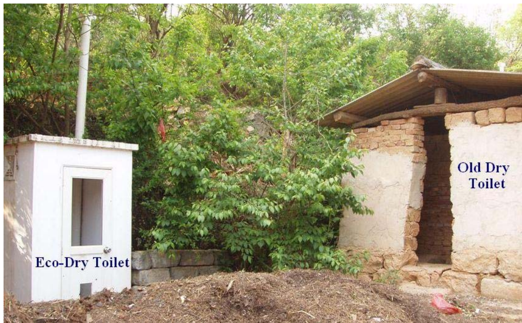
Figure 3-2 Old and New Toilet
