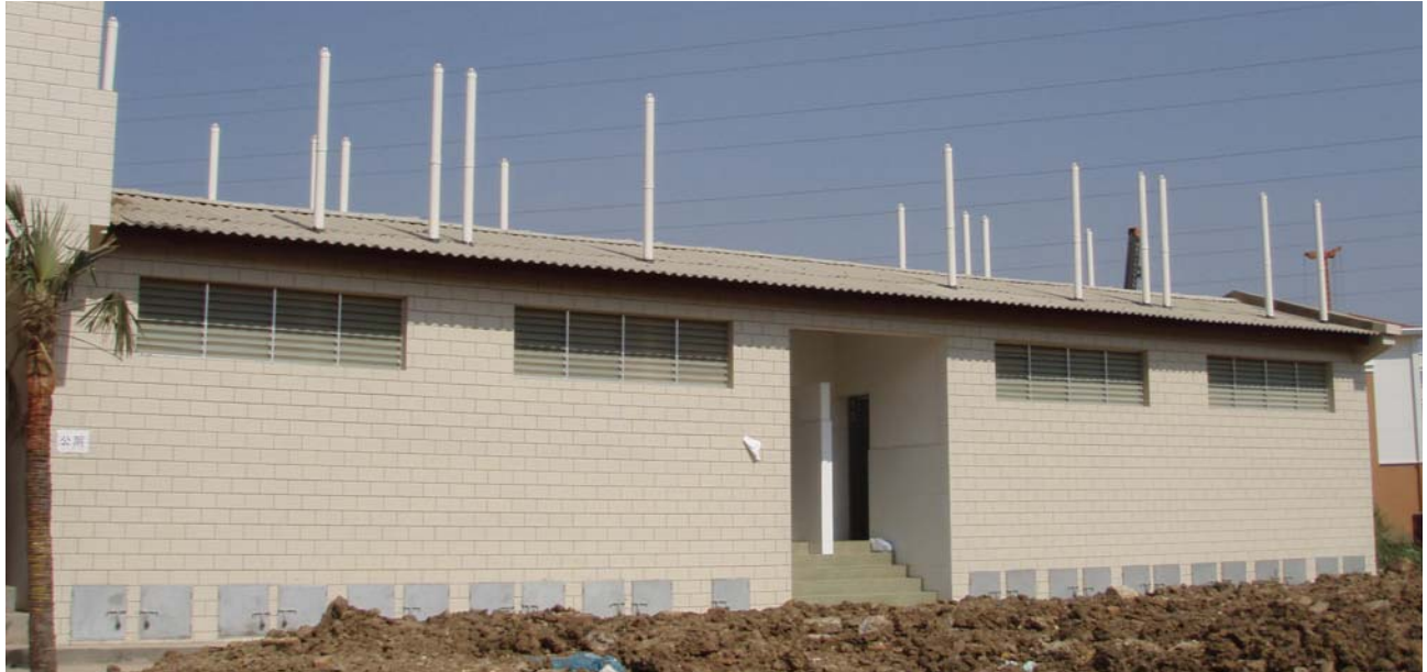
Figure 1-9 Public Eco-Dry Toilet (Photo by Miikka Ristkari in Guan Du district)
