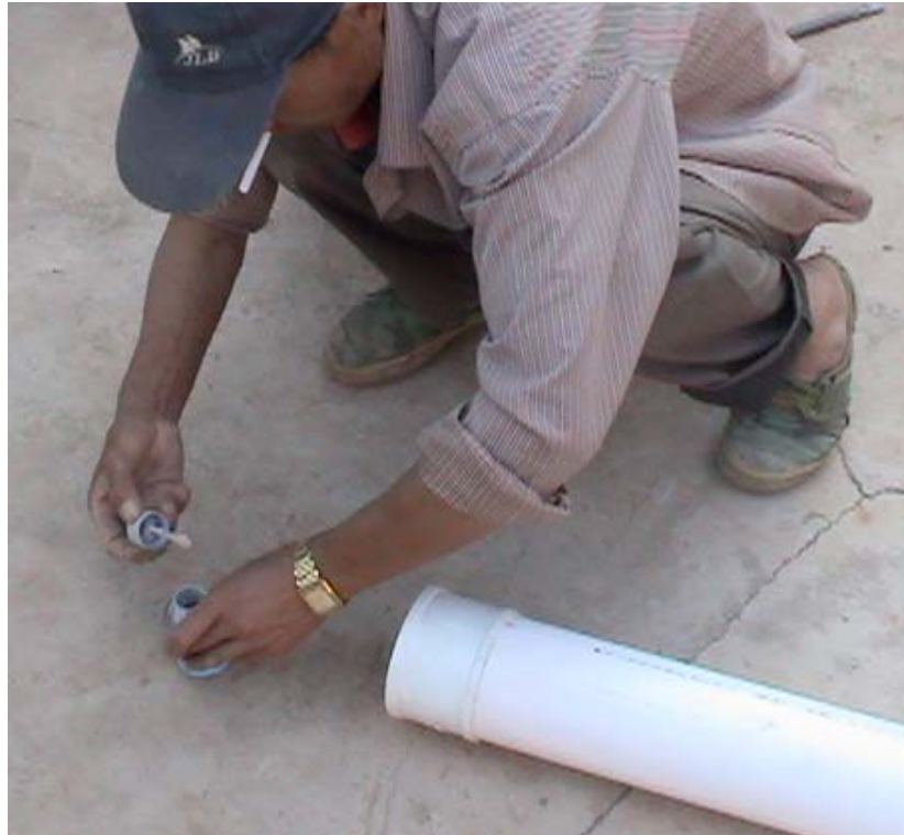
Figure 4-4 Adding Fly Net Between Ventilation Pipe And Ventilation Head
