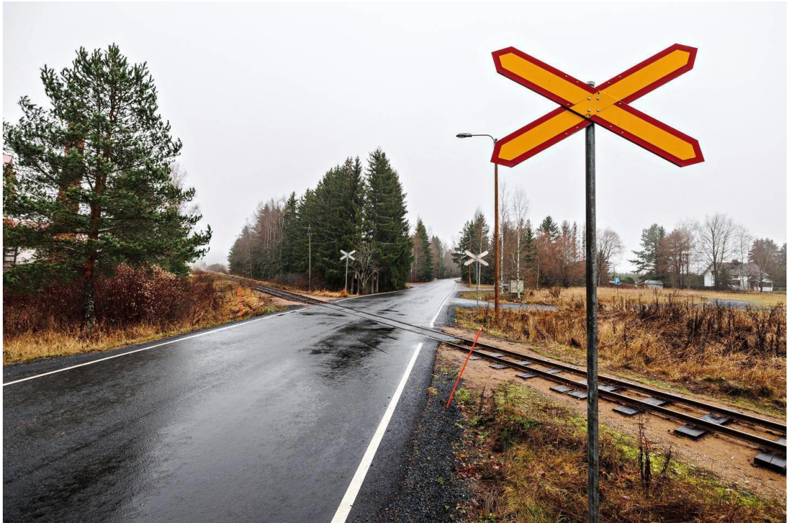
Figure 3. Un-guarded level crossing. (Pennanen, S. 2022)
