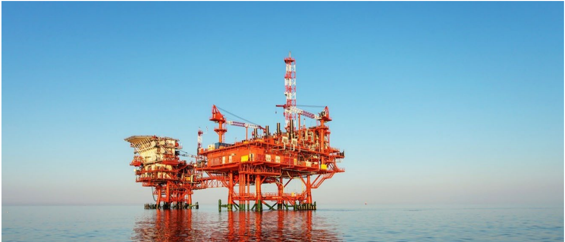
Figure 38. The sturdy, imposing oil rigs of the Baltic Sea between Helsinki and Tallin. They provide a blueprint for the hub's layout. There is something marvelous behind the industrial structure protruding from the calm sea (Entre 2015)
