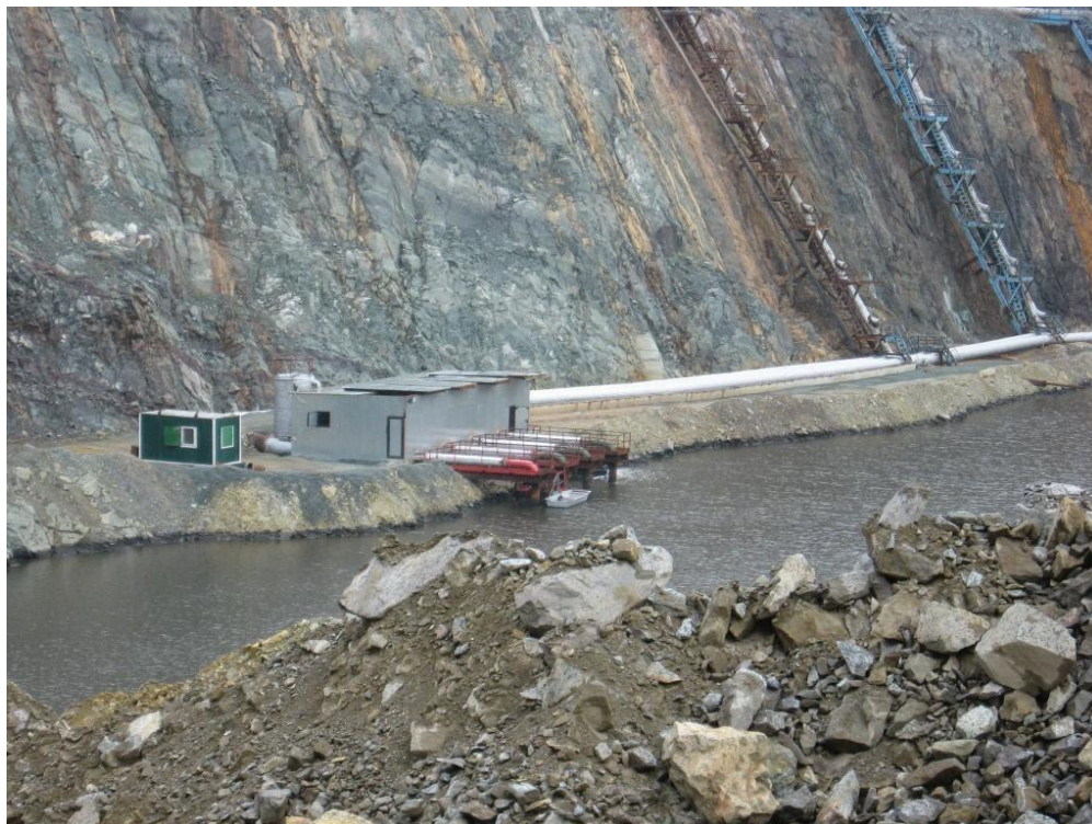
FIGURE1 6. Water treatment facilities of Gaisky GOK. /48/.
