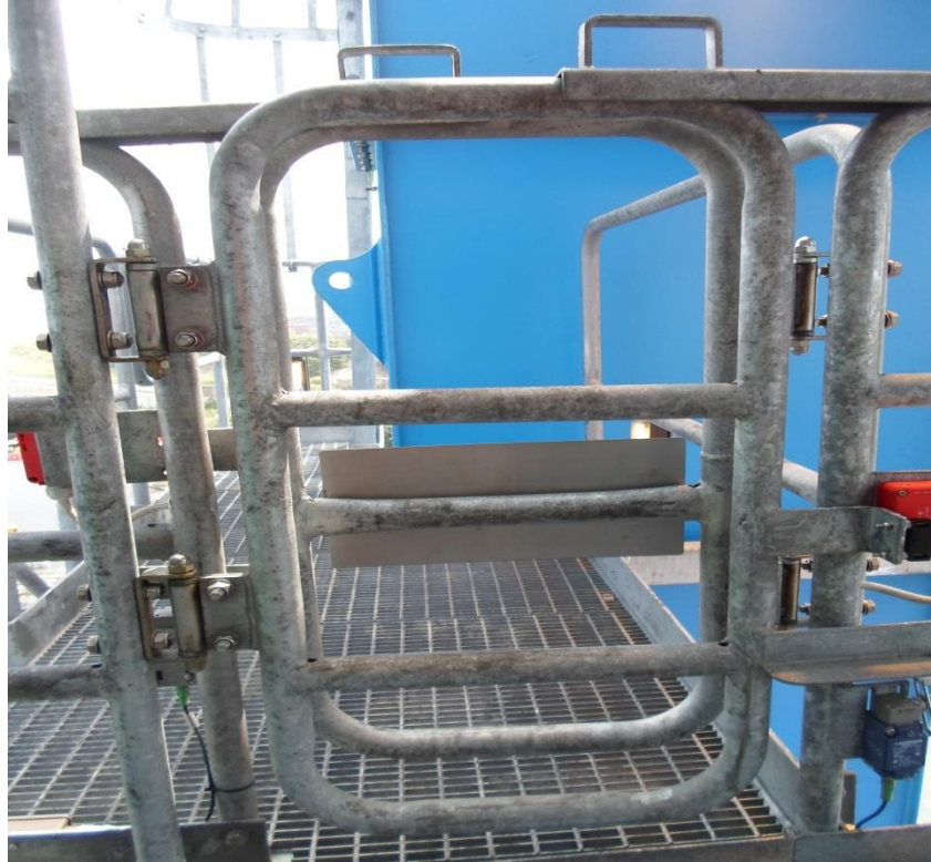
Figure 27 Gate aligned when trolley is at gate position
