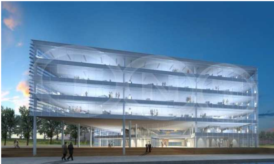
FIGURE 5. TNT Green Office /9/.
