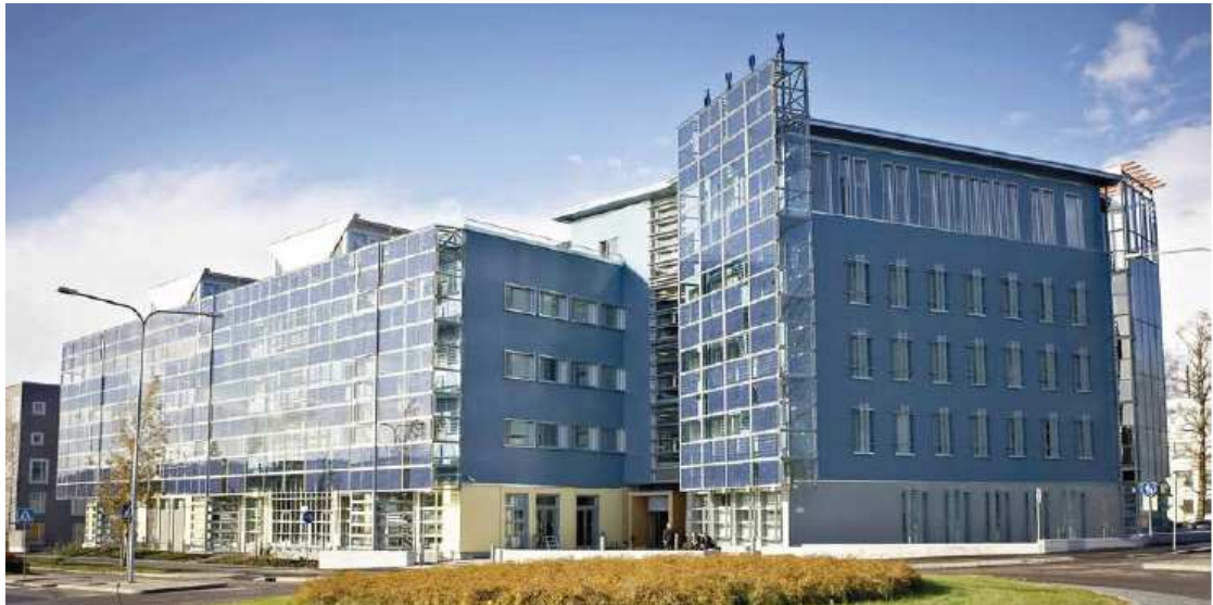
FIGURE 7. The Environment Centre building Ympäristötalo exterior /10, p.46/.
