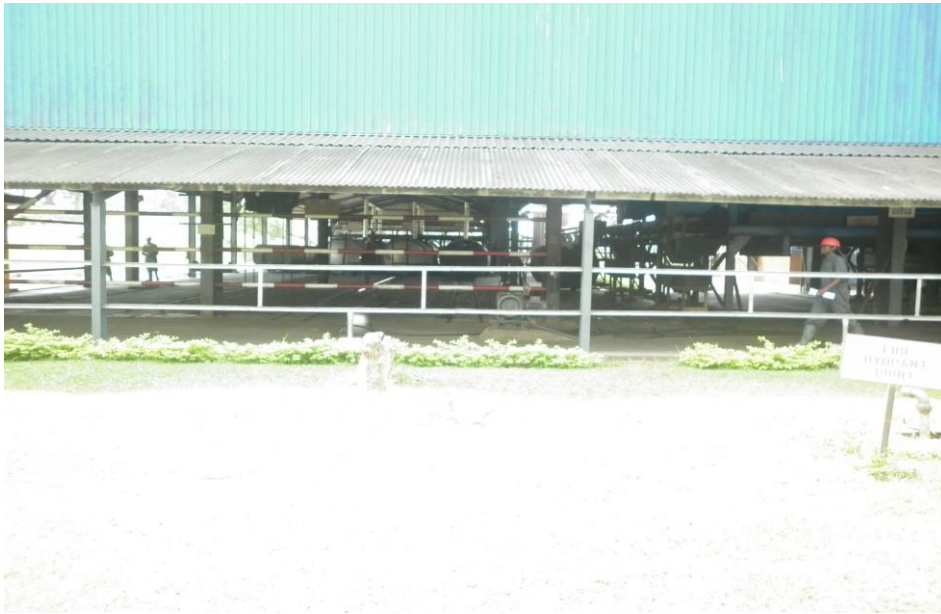
Figure 3. Back view of Plant area at TOPP.
