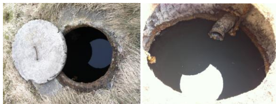
GRAPH 2. Wastewater tank at Mr K's summer cottage
