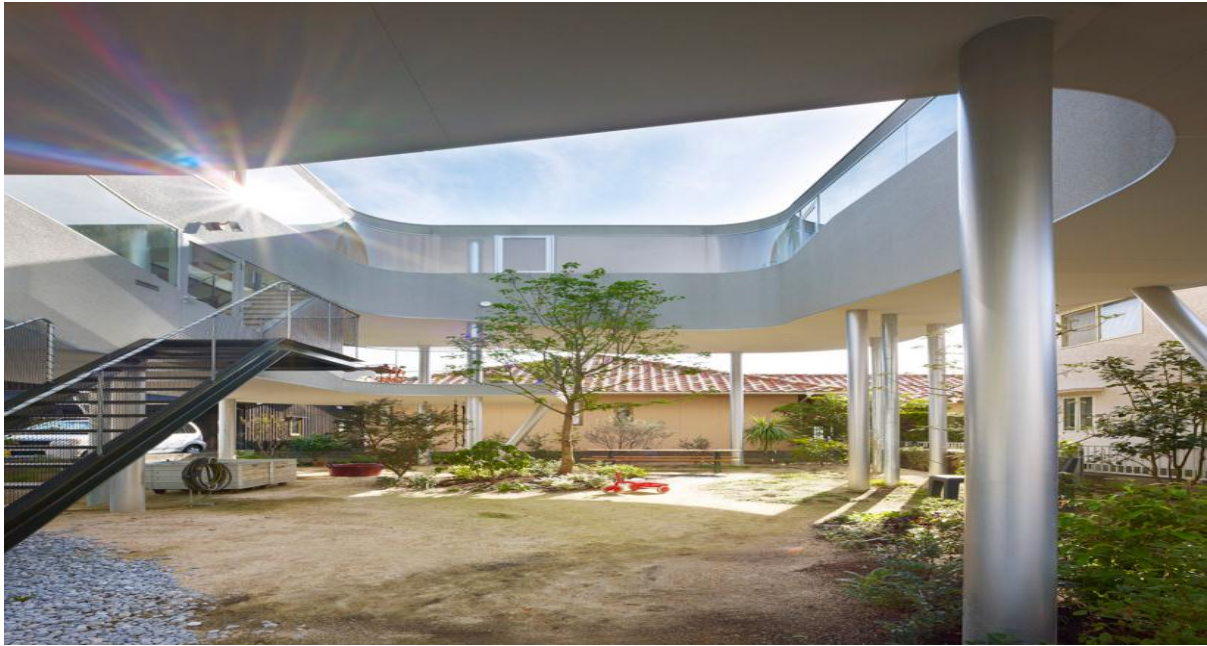
Figure 19: Polycarbonate (PC) is used here to make a roof for a house
