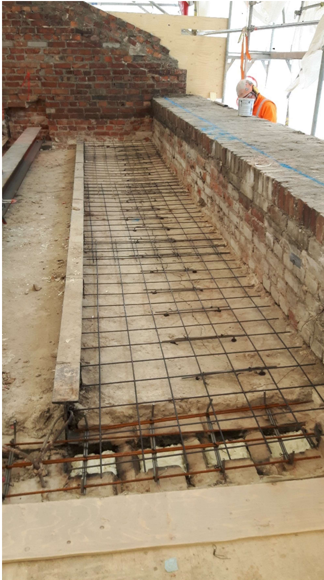
Figure 6. Repaired intermediate floor slab
