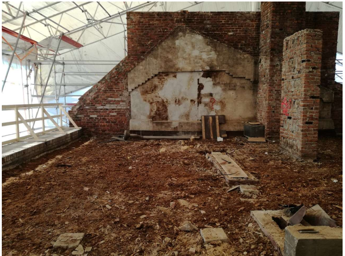
Figure 4. Demolished roof structure
