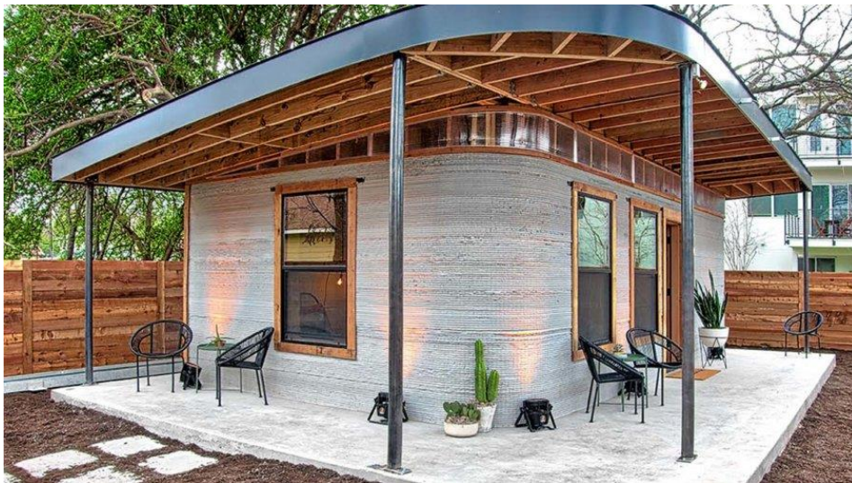
Figure 1. A 3D printed house in Austin, Texas [15]
