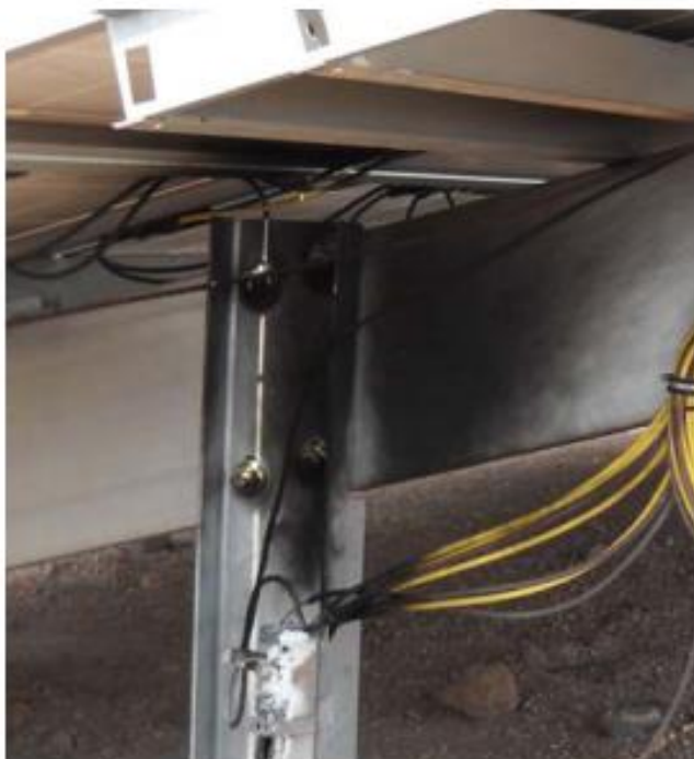
Figure 6 PV Panel Arc Flash
