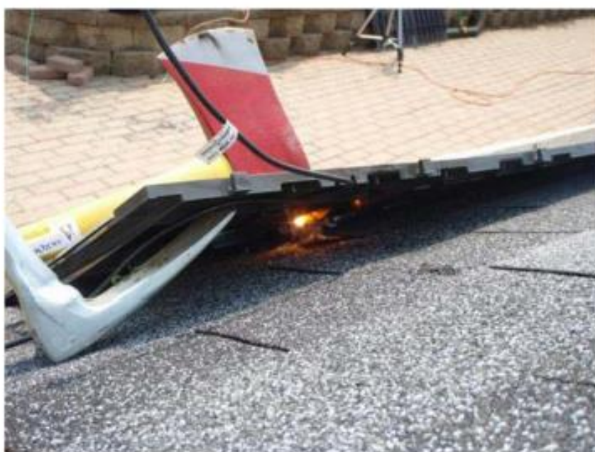
Figure 9 Arcing Caused by Penetration of PV Module
