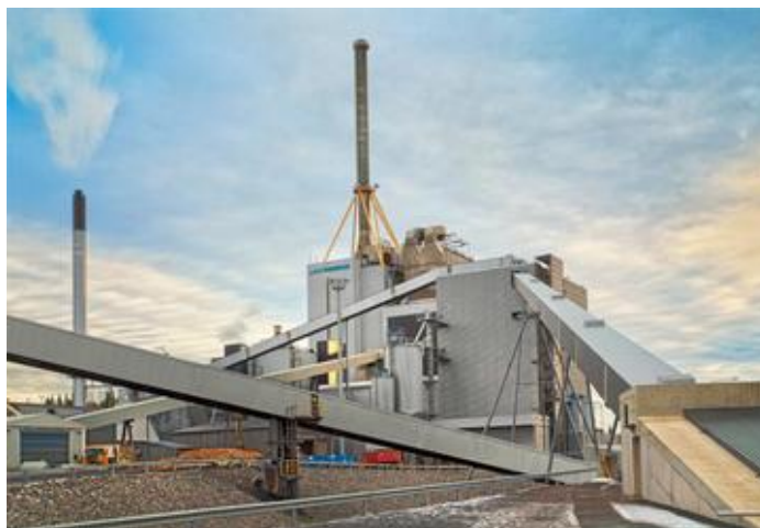
FIGURE 2. Lahti Energy's Kymijärvi II power plant (Lahti Energy 2011)
