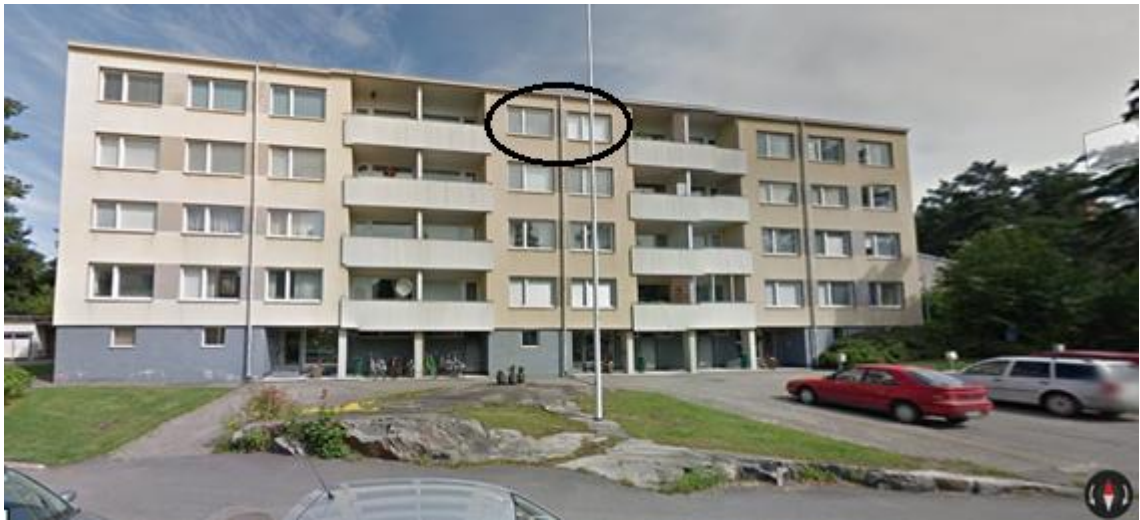
Picture 21: Example of an apartment building in Helsinki at Poutamäentie 7 facing directly south with large window area and has also sun exposure from east and west with no or little shading from trees. The circled windows belong to a 28 m 2 single-room apartment. One window is estimated to be 1.6 m wide and 1.2 – 1.3 m high. Owned by VVO / LUMO [43].
