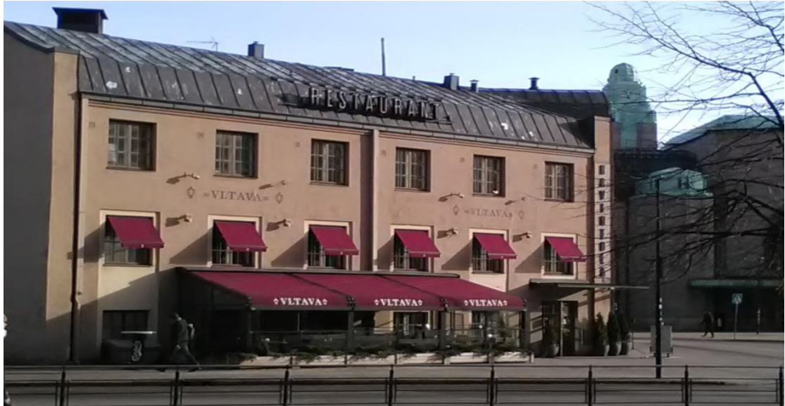
Picture 6: Restaurant Vltava at Elielinaukio in Helsinki has both slope and ornamental shapes in use. The slope model covers a terrace.
