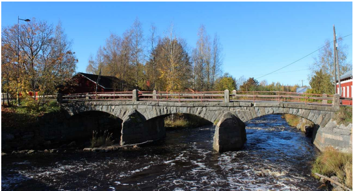
Figure 29. Pomarkku Bridge, October 2016. (WSP)
