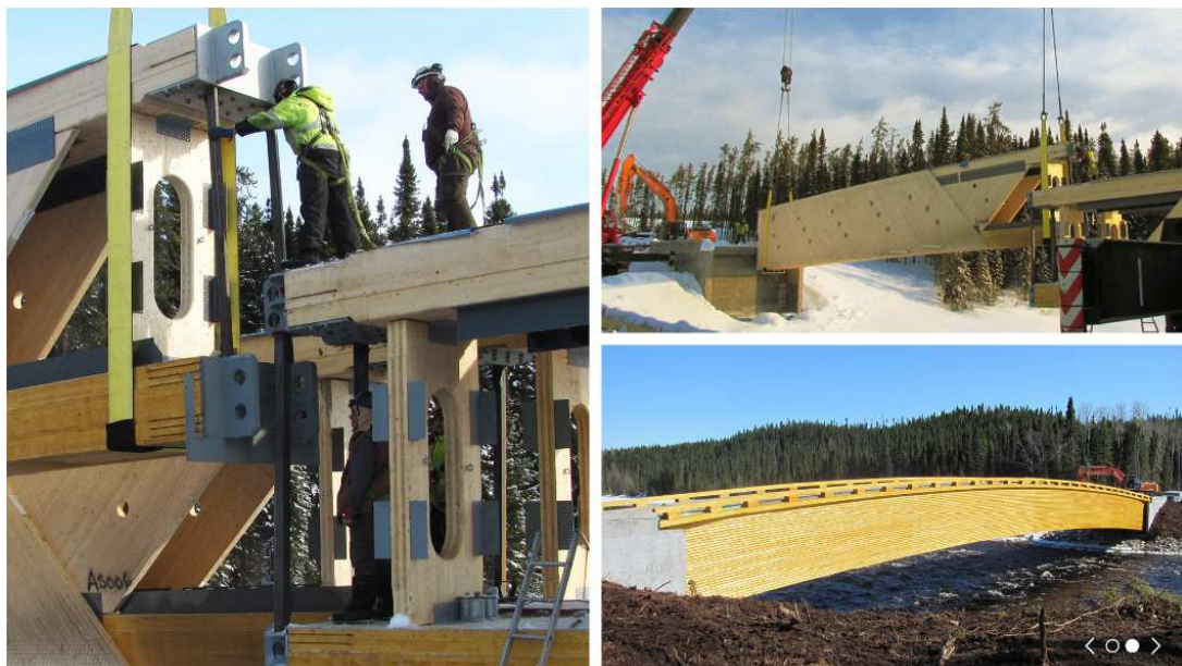
Figure 27. Macaisagi Bridge. ( http://nordic.ca )
