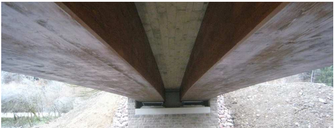
Figure 11. Birkbergbrücke, bottom view. (14)
