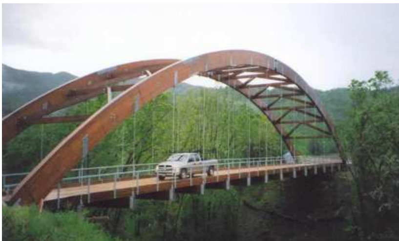
Figure 26. Hopland Casino Bridge. (22)
