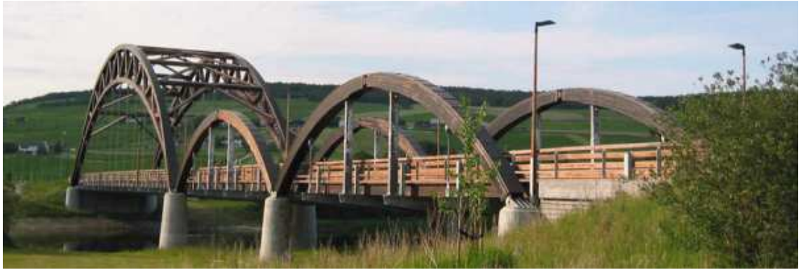
Figure 22. Tynset Bridge. (Photo: K.Bell)
