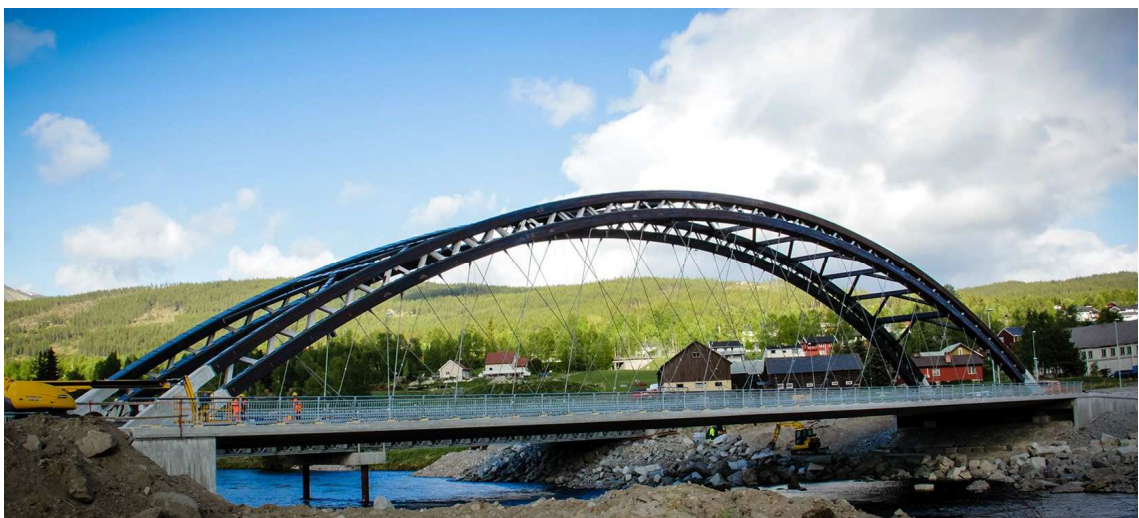
Figure 24. Steinen Bridge. (Photo: Kai Røen)
