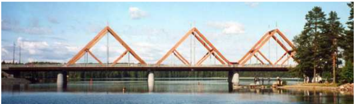
Figure 13. Vihantasalmi Bridge. (Photo K.Bell)
