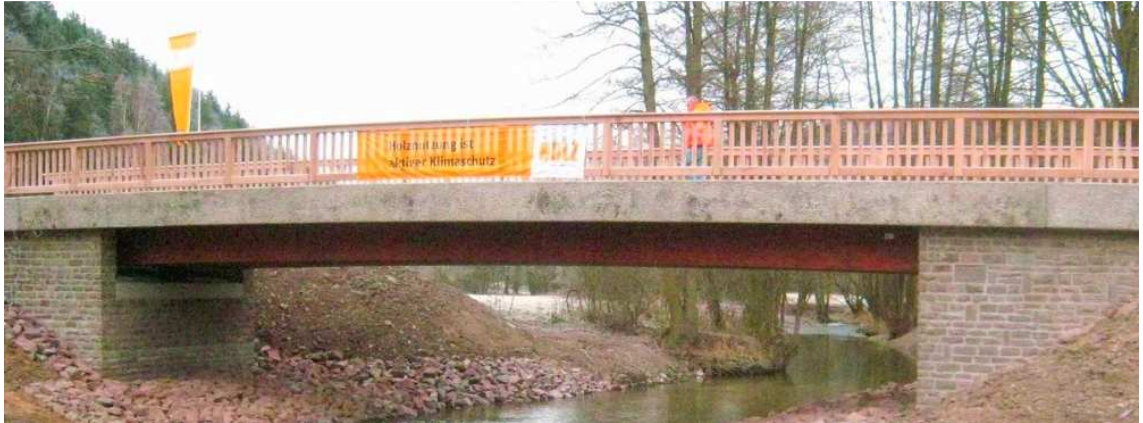
Figure 10. Birkbergbrücke, general view. (14)
