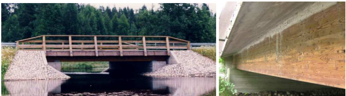
Figure 8. Kruununmylly Bridge. General view and deck detail. (13)
