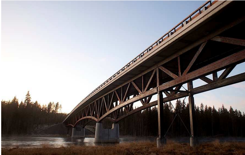
Figure 20. Kjøllsæter Bridge. (bridgeinfo.net)
