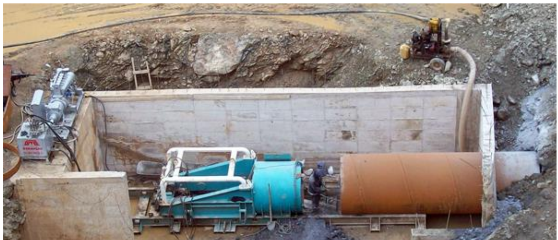
Figure 2.5 The pipe ramming process in action.
