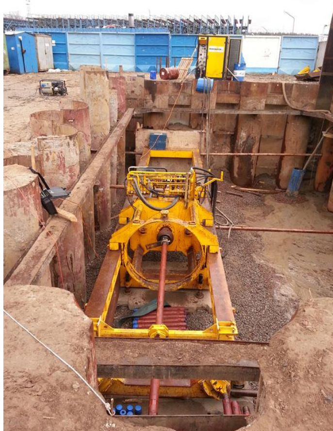
Figure 2.4 The pipe ramming machine.
