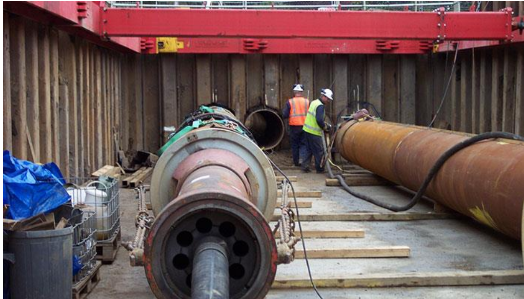
Figure 2.6 The preparation for pipe ramming.
