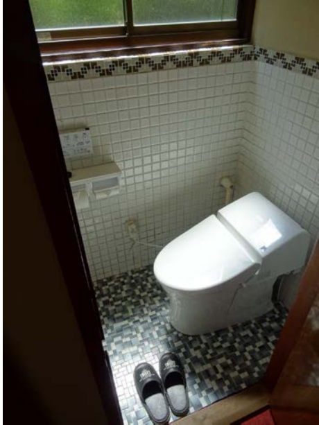
Figure 12: Renovated Toilet (Pallaspuro 2016)
