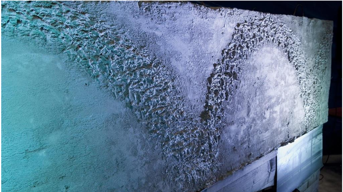
Figure 15. The wall printed on 3D printer by FIMAttec (99)
