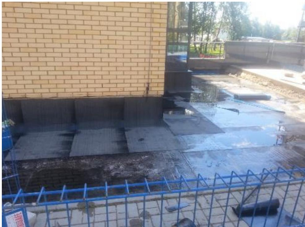
Figure 36. Building walls waterproofing with Icopal H
