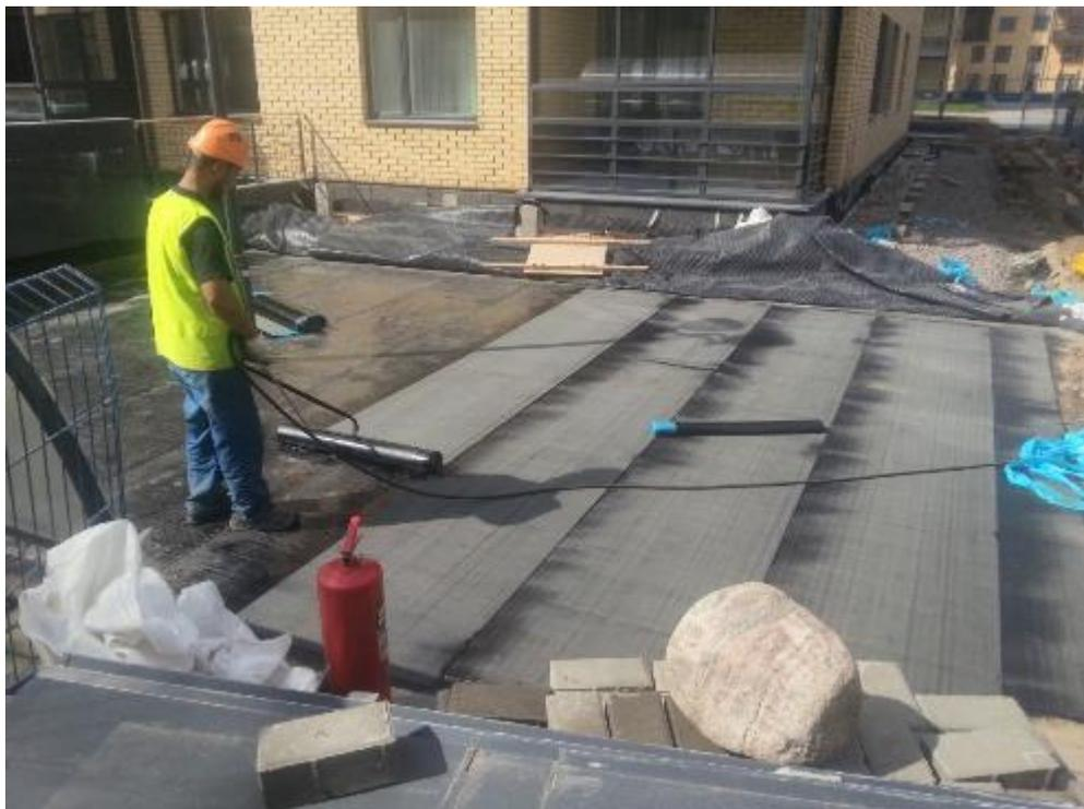
Figure 35. Roof waterproofing with Ultratap membrane slope (1:70)
