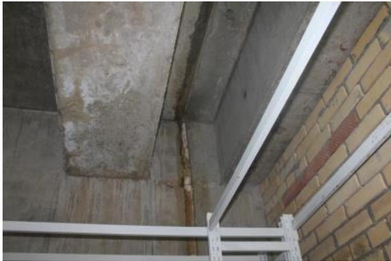
Figure 26. Deformation joints
