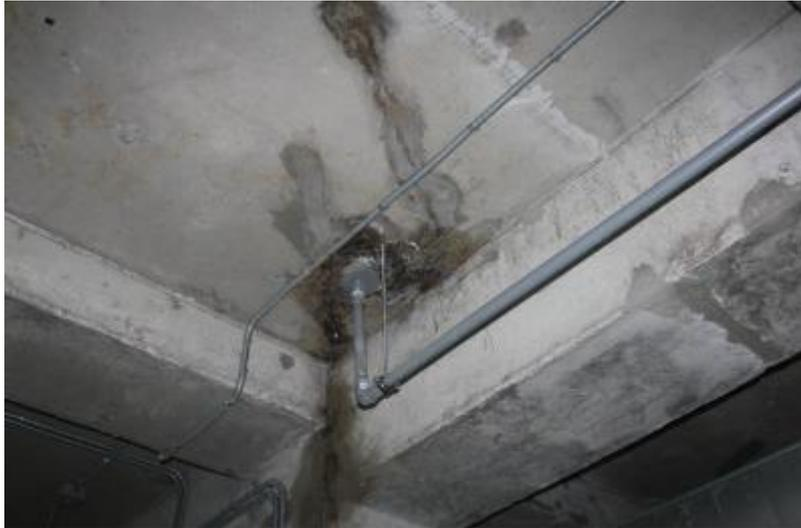
Figure 25. Water filtration through drainage system
