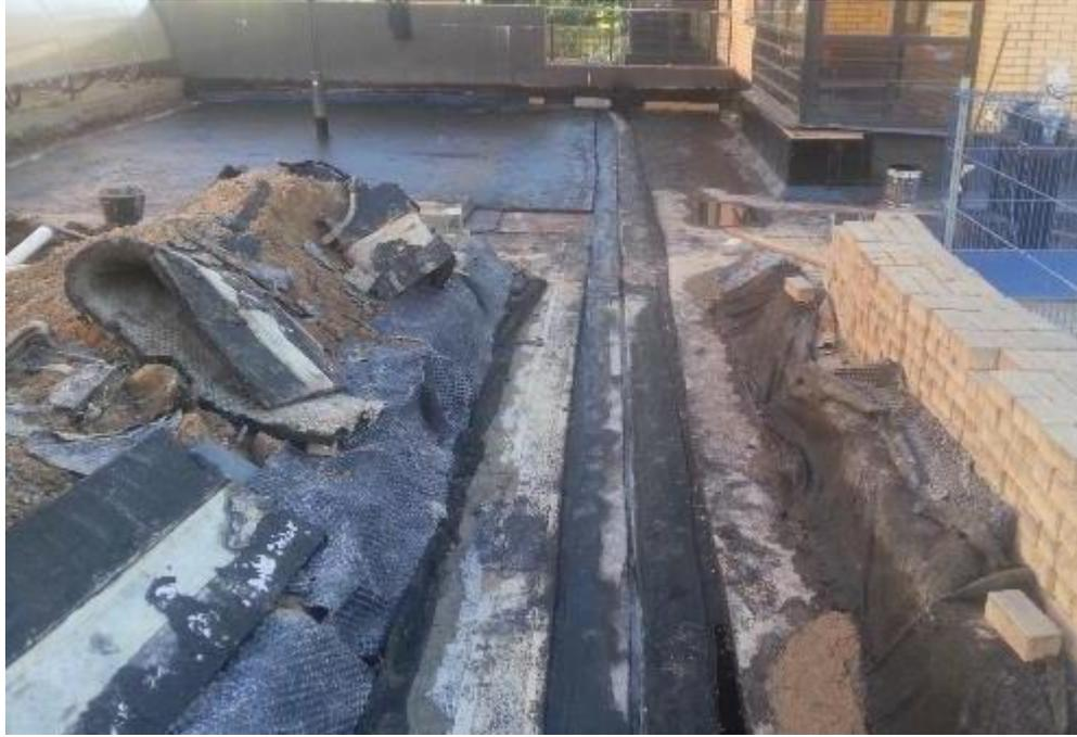
Figure 34. Removing of roof covering
