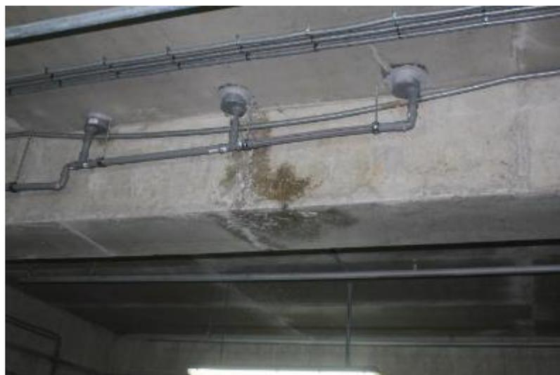
Figure 24. Water filtration through drainage system
