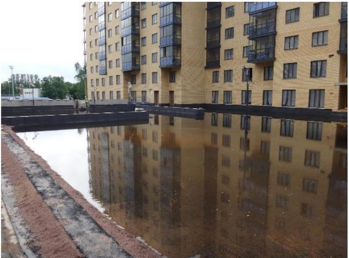
Figure 42. Waterproofing testing
