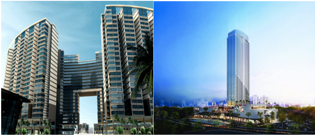
Picture 4: Model of Waterfront City (in the left) and Vinhomes Riverside Haiphong (in the right) (Duy 2011 & Thanh 2016).
