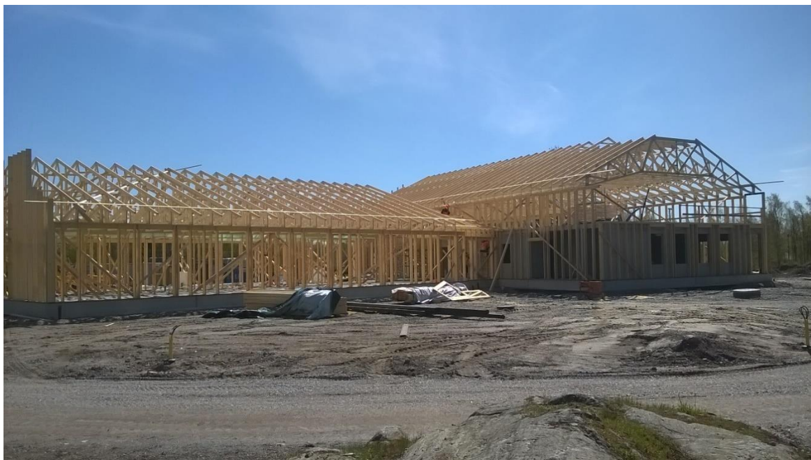
Figur 87. Betongplattan gjöts under bar himmel.
