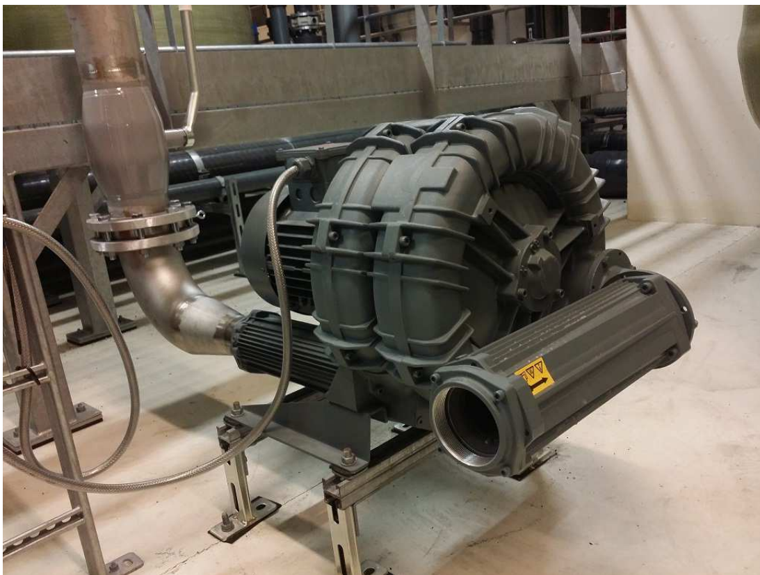
Figure 6 Air compressor used in rinsing.
