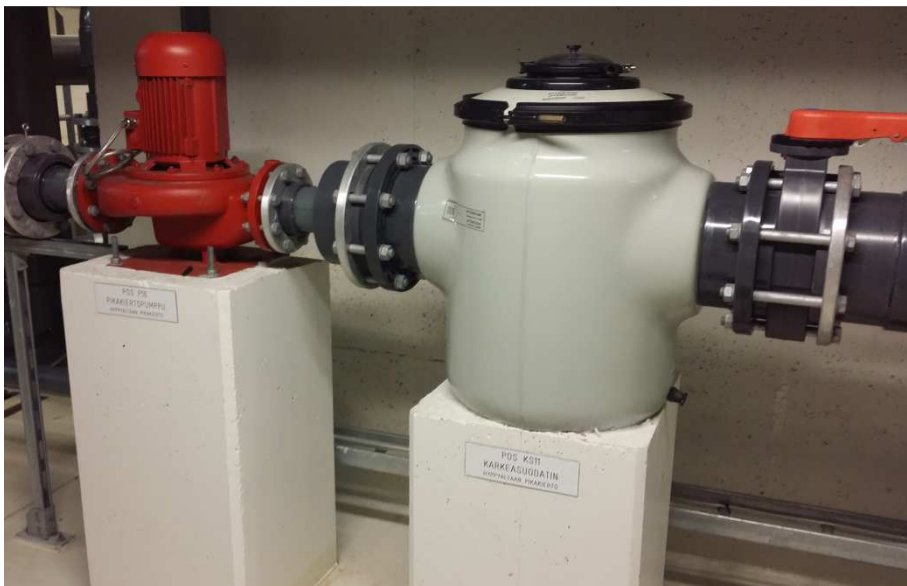
Figure 2 Red circulation pump and the gray basket filter.
