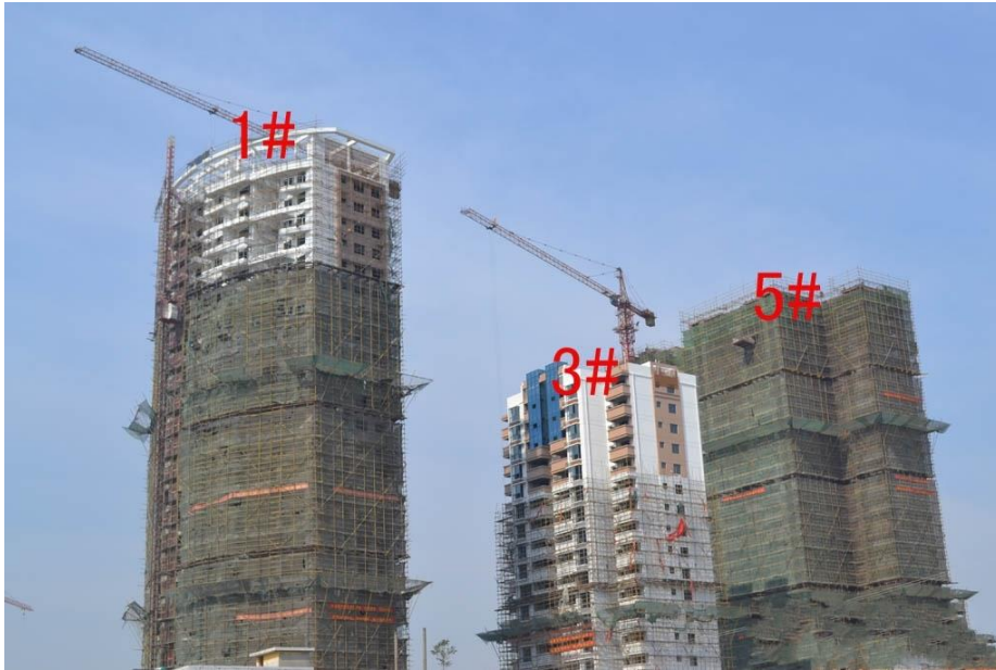
IMAGE 8. The construction of XinDe Square in April, 2011 (House.La.Xafc 2011)
