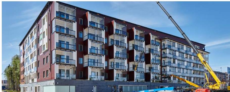
Figure 16. PuumERA project under construction, [70]
